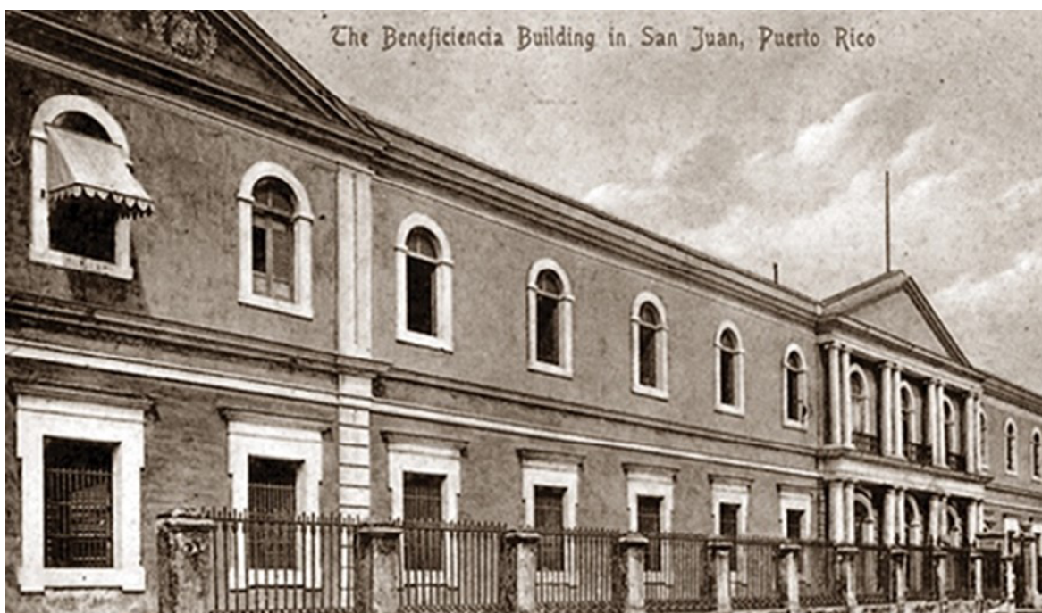
The Beneficiencia Building in San Juan Puerto Rico. Tarjeta Postal (circa 1905).
